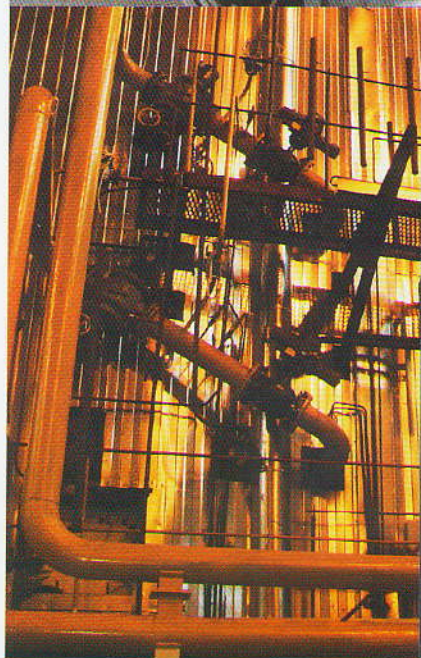
8 waste heat boilers (KUV-33) after 8 General Electric MS-5001 (26 MW) at 200 MW power plant, Vankor Oil Field, Russian Federation
