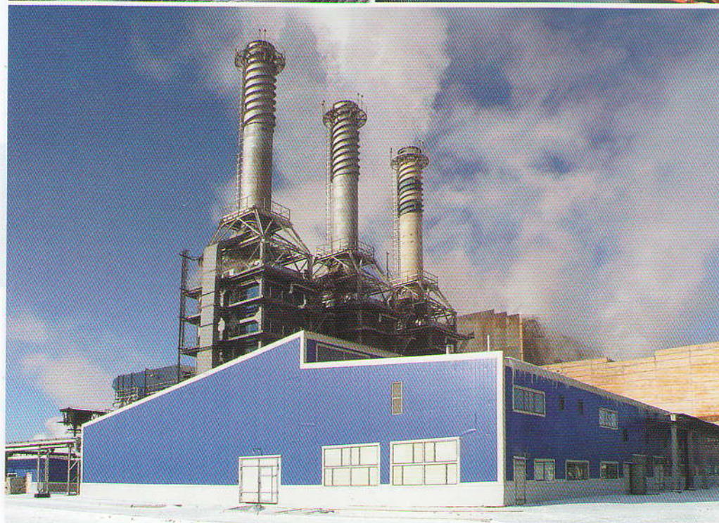
GTE-50 (3 x 15 MW) + KUV-30 (3 waste heat boilers), Kzyl-Orda, Kazakhstan
